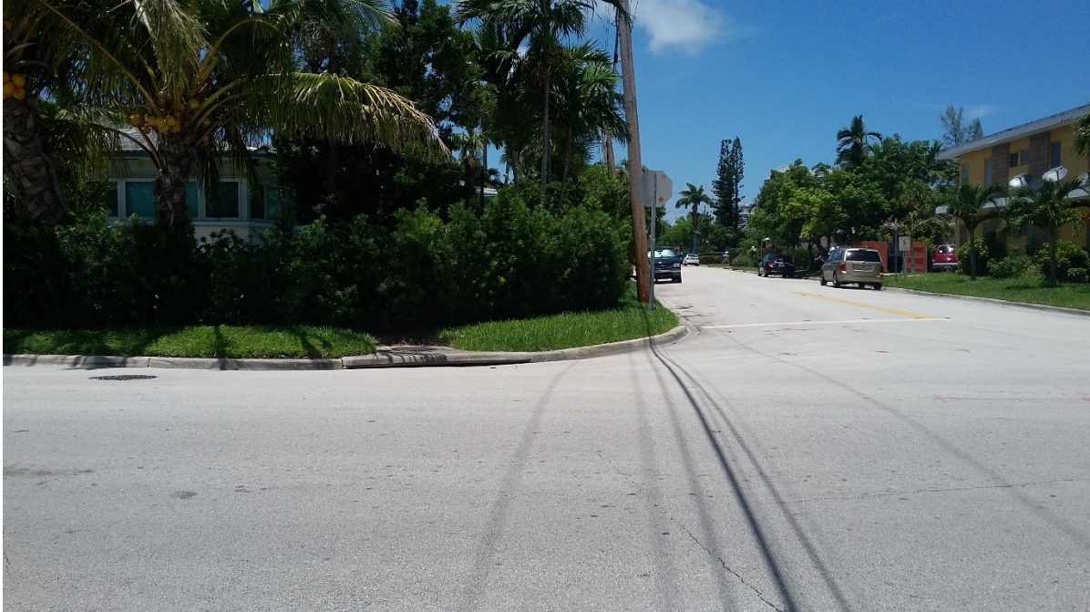
FPL POLES BEHIND BACK OF CURB, ABBOTT AVENUE AT 91 ST STREET
