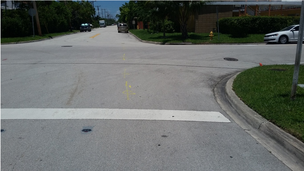
ABBOTT AVENUE AT 91 ST STREET (LOOKING NORTH)
