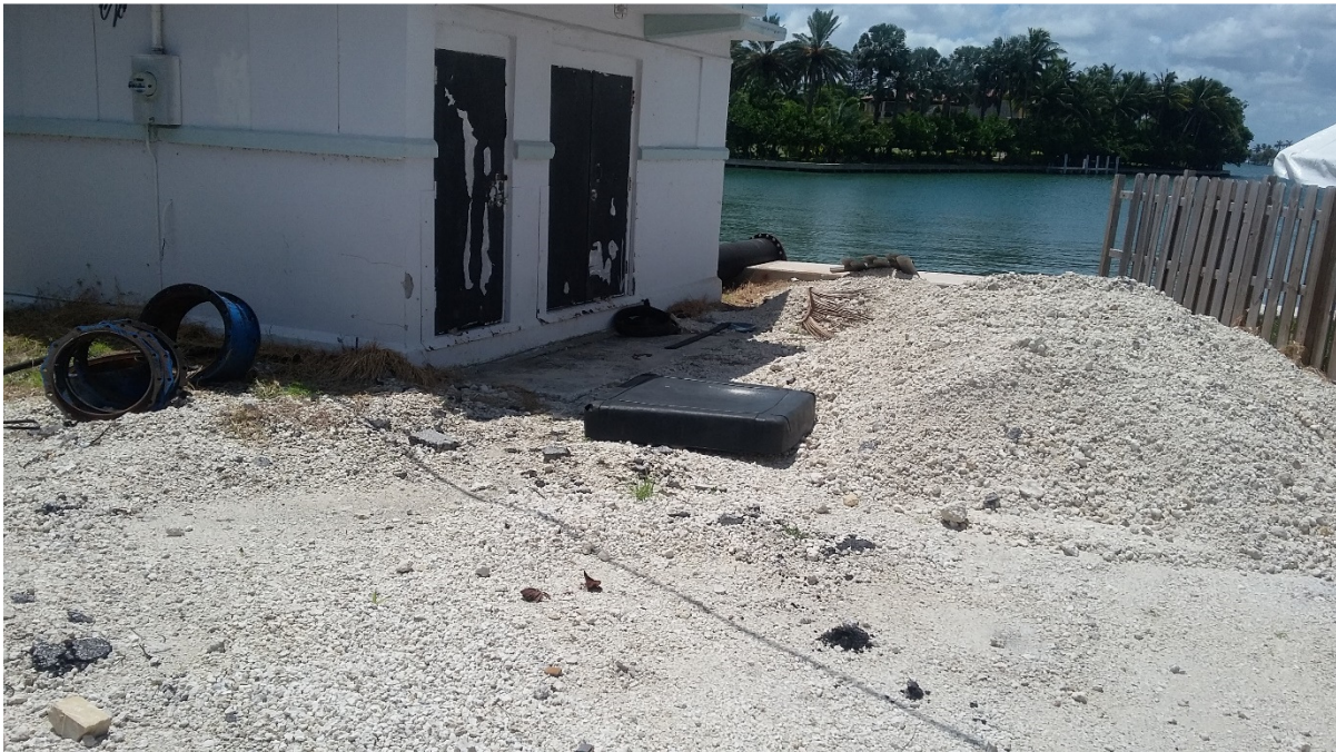
EXISTING PUMP STATION AT 92 ND STREET, CURRENTLY NOT IN SERVICE
