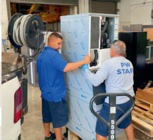
Maintenance Supervisor Josvani Iglesias and Carlos Duarte assembling the new ice machine in the Public Works Garage.
