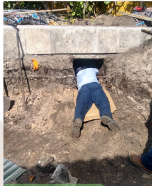
Water & Sewer Maintenance Worker Curtan Turner repairing a backyard residential waterline.
