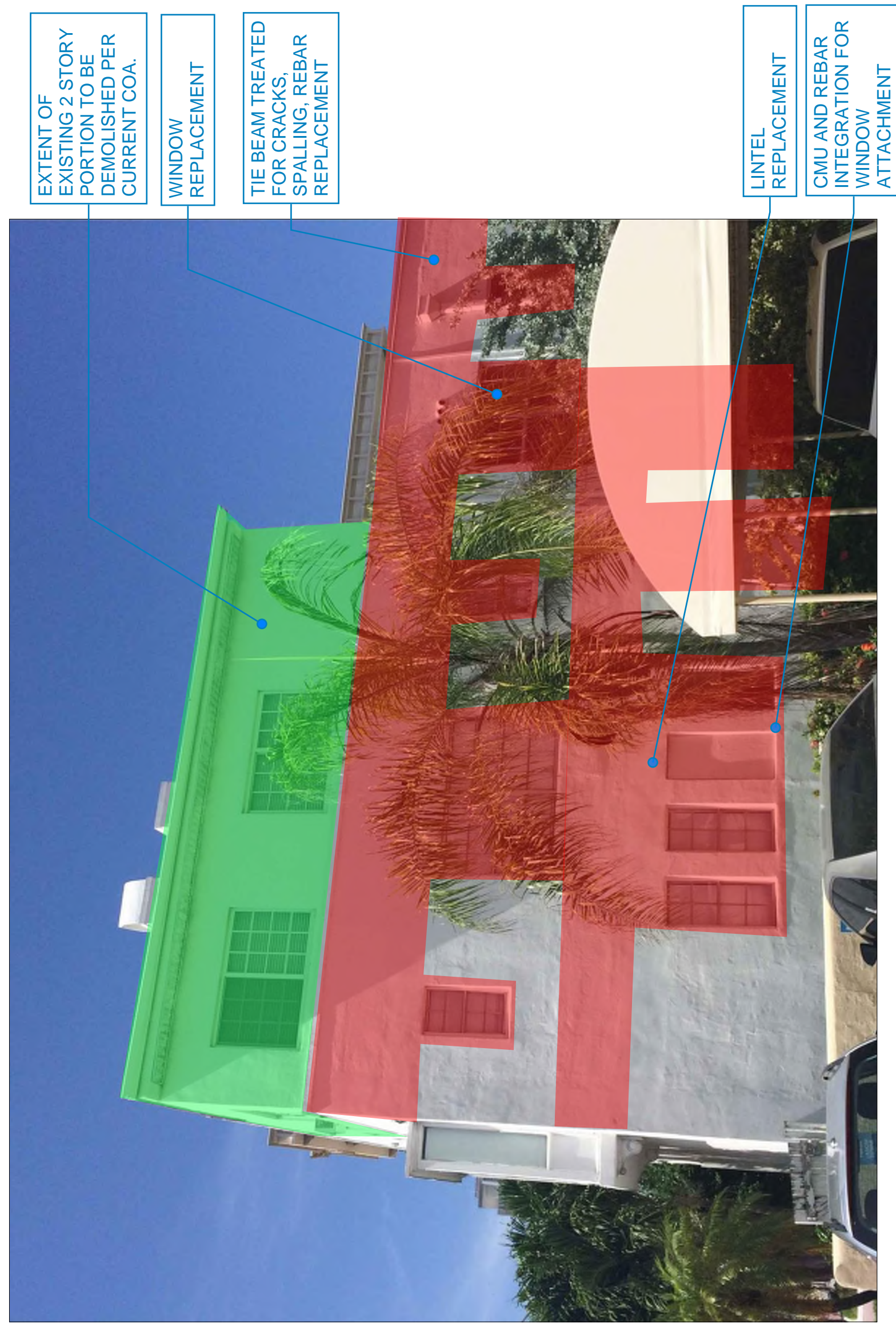
3 SOUTH EXTERIOR ELEVATION
