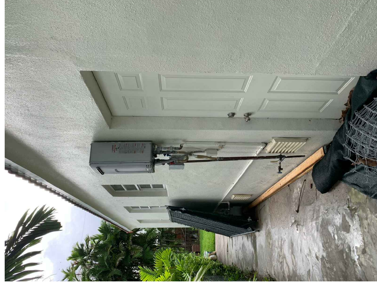
SIDE NORTH FACADE
