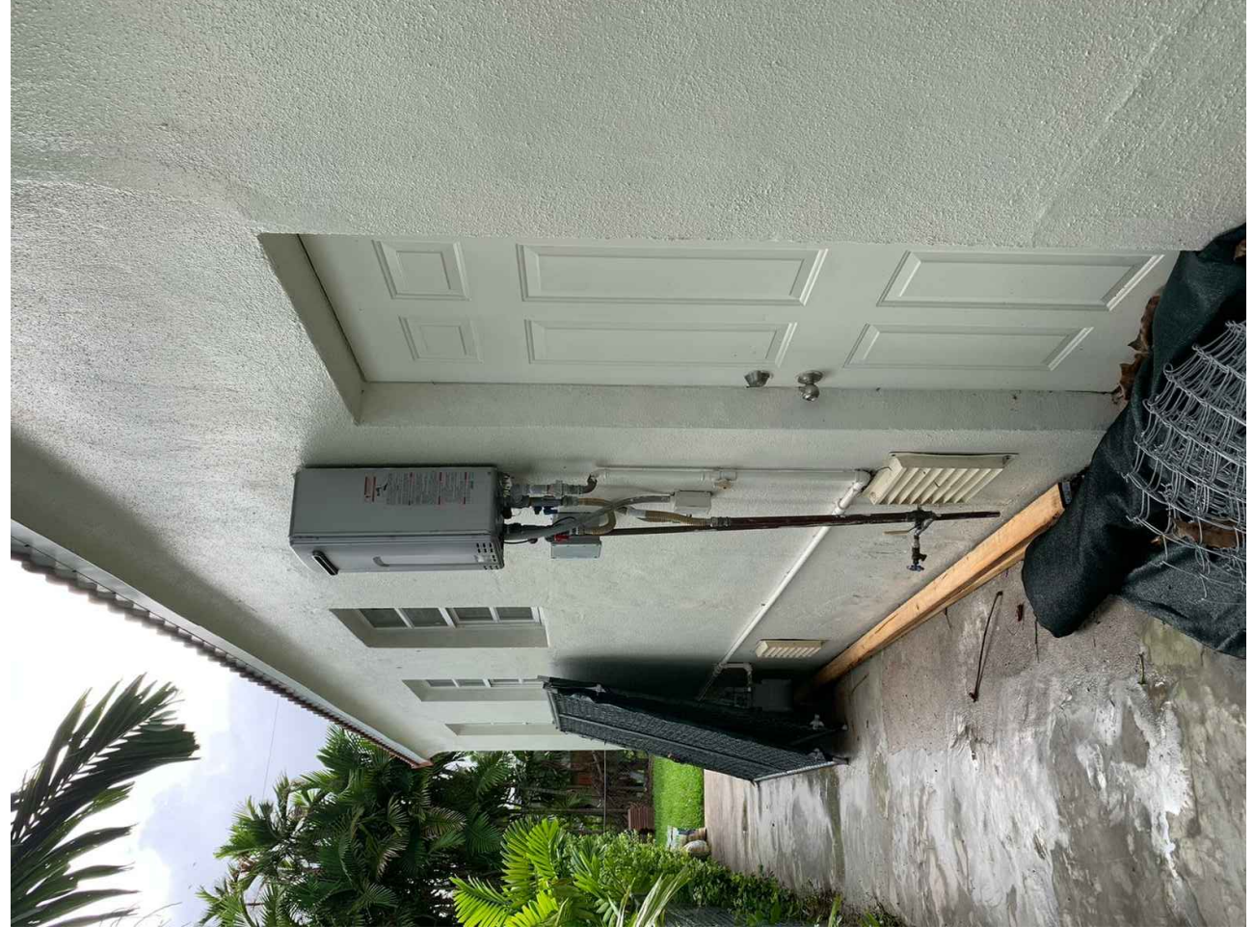
SIDE NORTH FACADE
