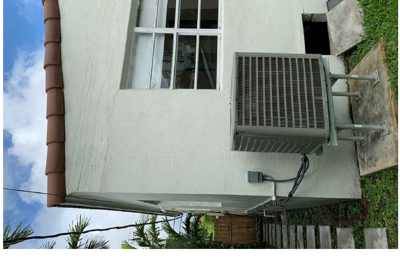
SIDE SOUTH FACADE
