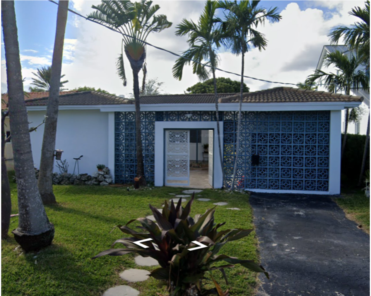
9524 Carlyle Avenue Miami-Dade County Property Appraiser Google Street View
