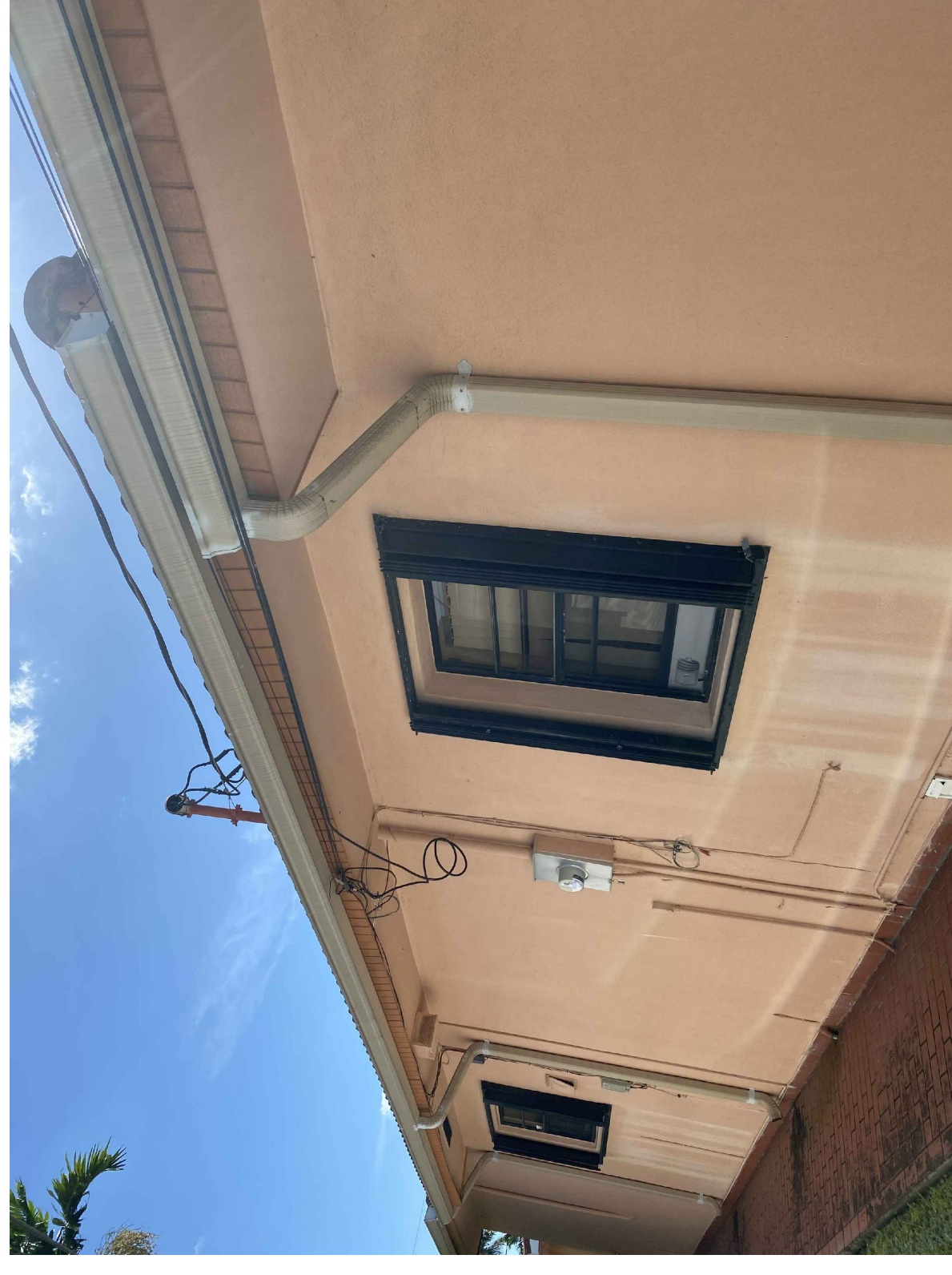
SUBJECT PROPERTY NORTH ELEVATION
