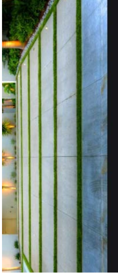
Concrete driveway with grass inlay
