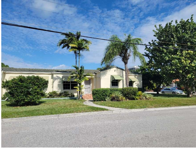
VIEW FROM 94 TH STREET
