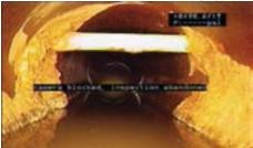
Inspection camera shows a pipe section that is blocked and damaged.
