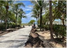
The department also started rebuilding the 90th Street Beach End walk path and nature area. Construction began on June 1st and will be completed this summer. The work consists of replacing the original damaged pavers, adding irrigation, adding turtle friendly lighting and improving the overall experience for town residents and visitors.
